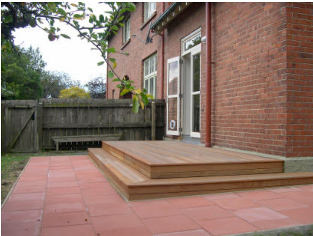
The Vicarage Kitchen/Dining Room is nearly finished
